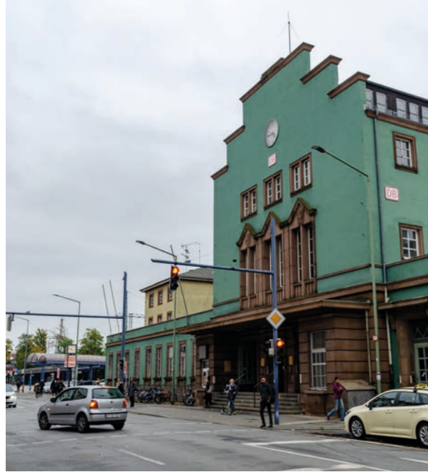
Haupteingang Main entrance
