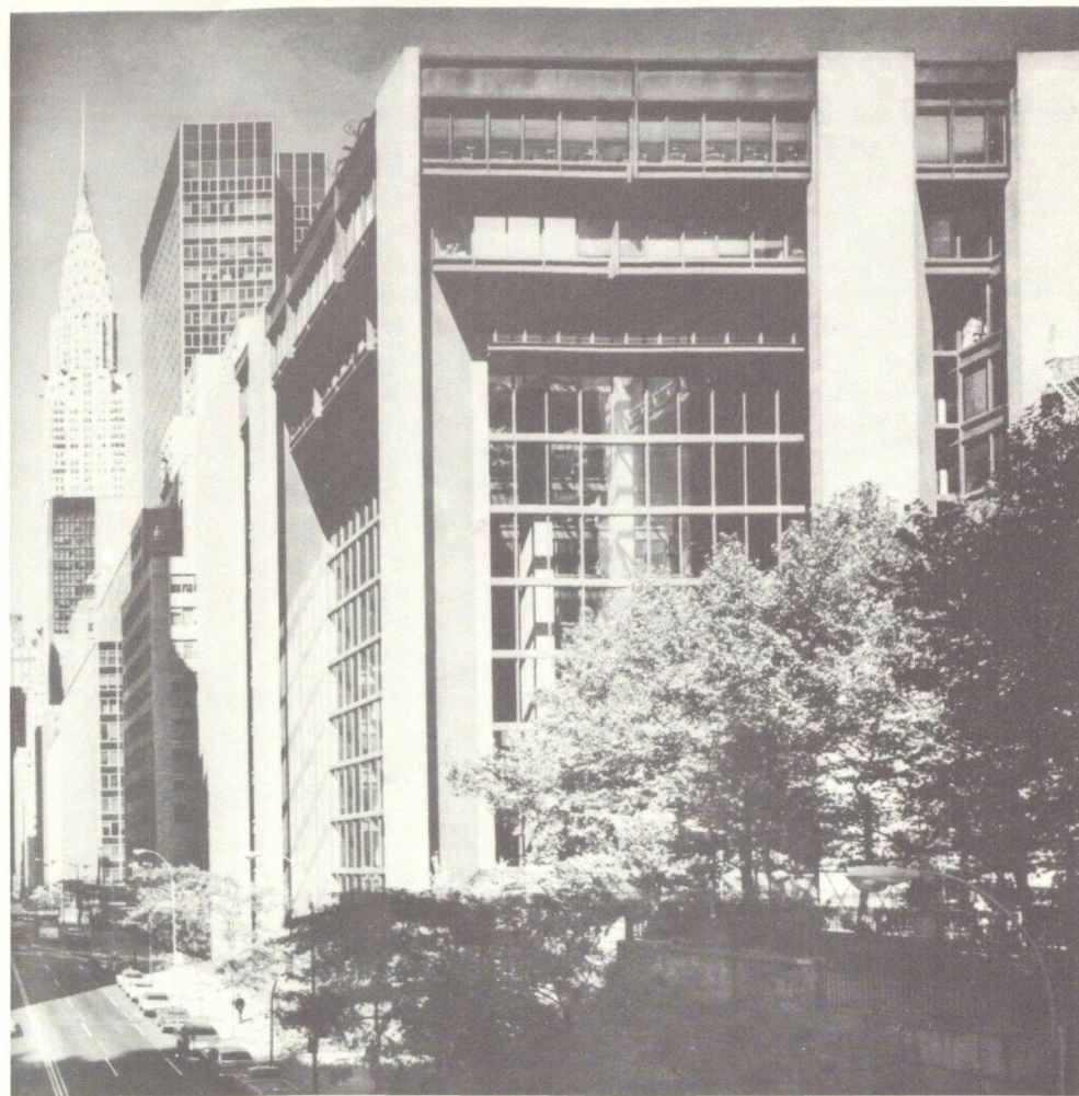
The Ford Foundation Headquarters, New York 1963; Fassade
